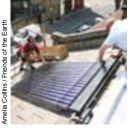
As well as making electricity, the sun's heat can be used to heat water in homes and commercial buildings. Solar hot water systems – sometimes referred to as solar thermal – are usually fitted on a roof with liquid-filled panels or tubes collecting heat in sunlight. These connect to a hot-water storage tank.
